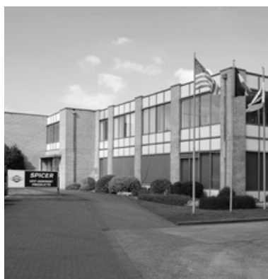
Dana Brugge Facility, Belgium
